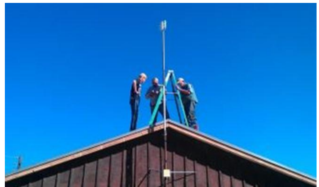
Steve, Dean and Val installing the Wi-Fi
